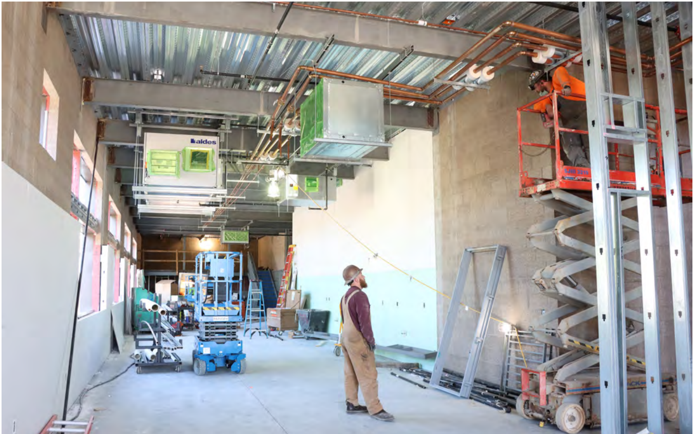
Roosevelt HS Phase 4 Construction, July 13, 2021
