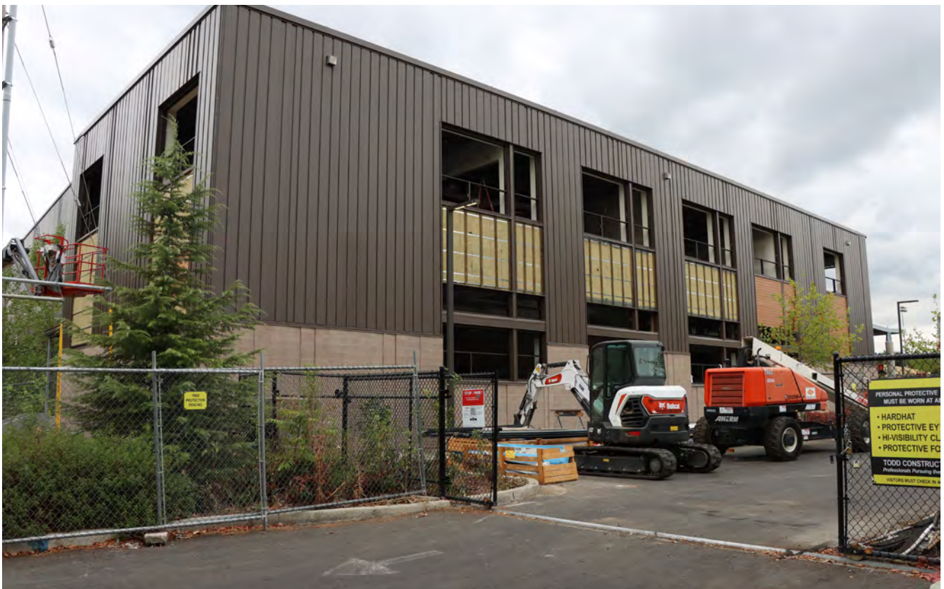
Roosevelt HS Phase 4 Construction, October 6, 2021
